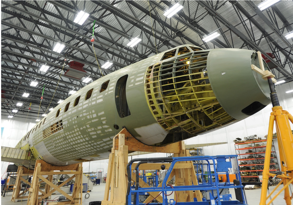
Lufthansa restoration in the Auburn-Lewiston Airport Hangar (Ralph M Pettersen photo)
